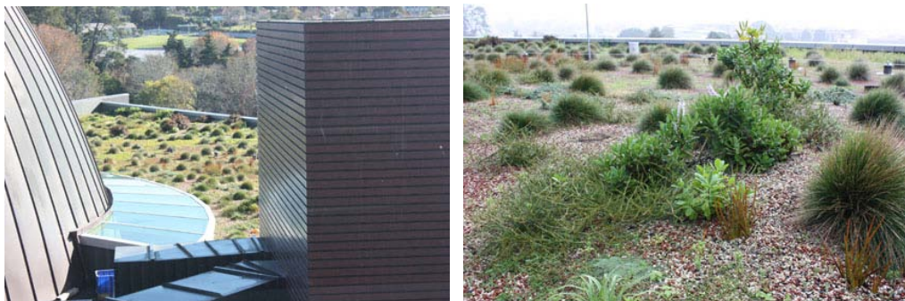
Figure 1a and 1b: The Waitakere Civic Centre living roof in June 2010 (mid winter) viewed from the adjacent building and showing the diversity of plant growth forms from tussocks ( Festuca coxii ) and spikey orange irises ( Libertia peregrinans ) to tangled ground covers ( Coprosma acerosa ) and dense mounds of NZ hebe ( Hebe obtusata ).
