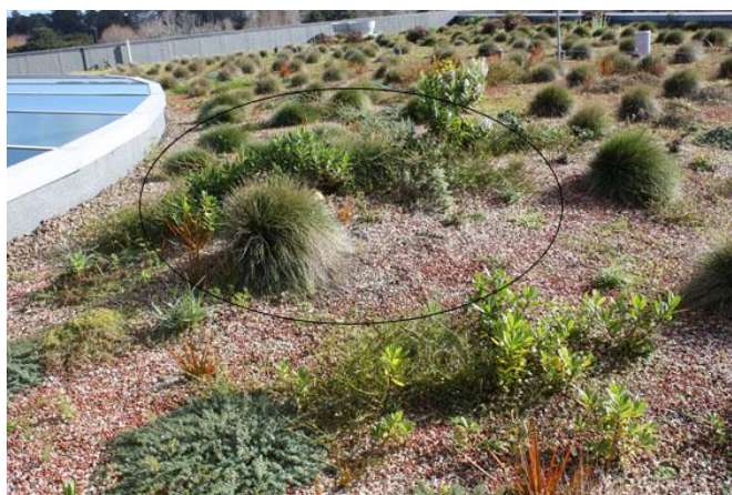
Figure 4: Mound (identified by black circle) created on WCC living roof showing different plant species able to survive in the deeper soil and shading opportunities provided by the taller plants and the associated micro-habitats.
